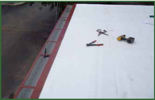
New pre-painted metal gutters are attached to the wood.
