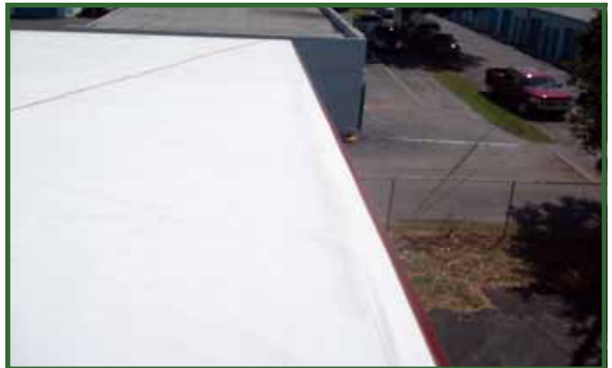
New edge metal is installed to complete the system.
